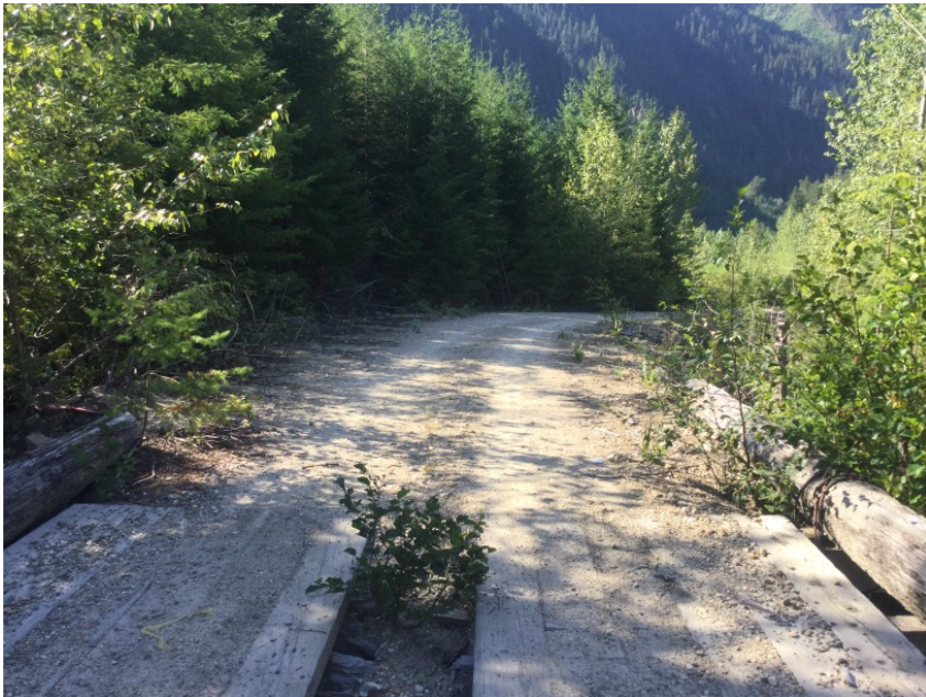
Left Approach Facing Away From Bridge
