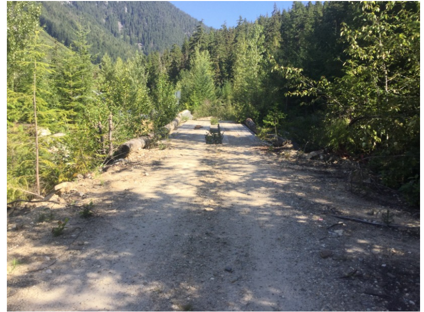
Left Approach Facing Bridge
