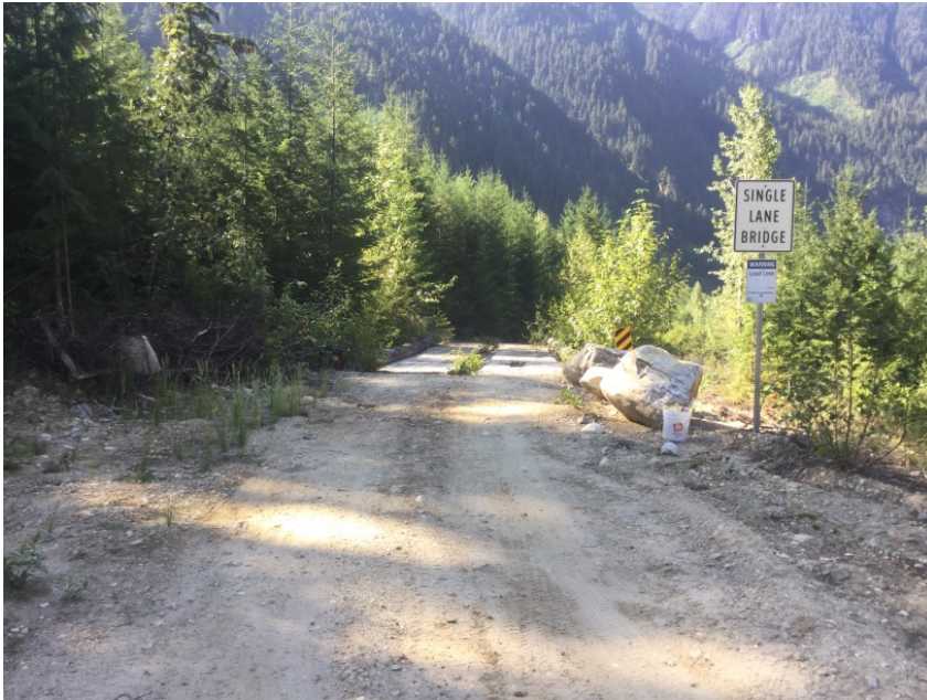
Right Approach Facing Bridge
