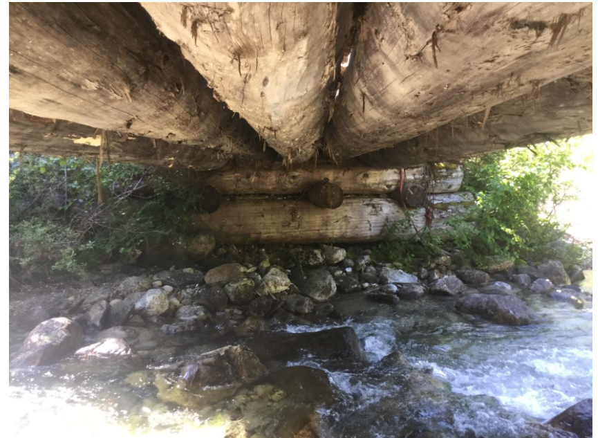
Left Bank Abutment
