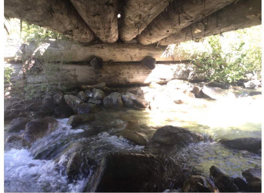
Right Bank Abutment
